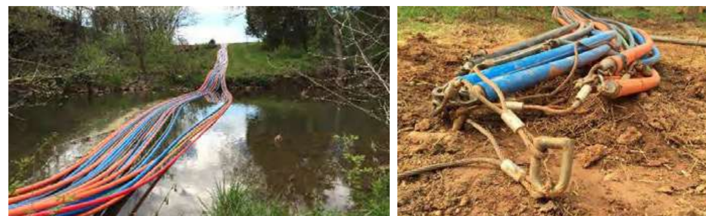
EXAMPLE: TWENTY 2" DUCTS INSTALLED UNDER A FIELD, A RIVER AND A GOLF COURSE – 800 FT
