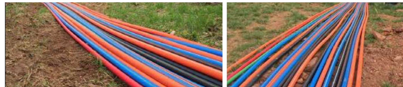
EXAMPLE: TWENTY 2" DUCTS INSTALLED UNDER A FIELD, A RIVER AND A GOLF COURSE – 800 FT
